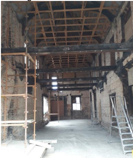
Stripped out Council Chamber
