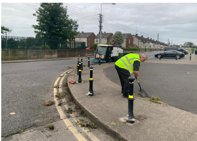
Weed clearing at Ballsgrove
