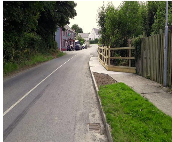
Dromin Footpath after works
