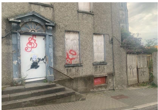
Graffiti Removal Duke Street Drogheda –Before
