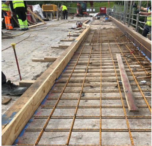
Upstream South elevation footway shuttered
