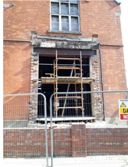
Dismantled Bay Window
