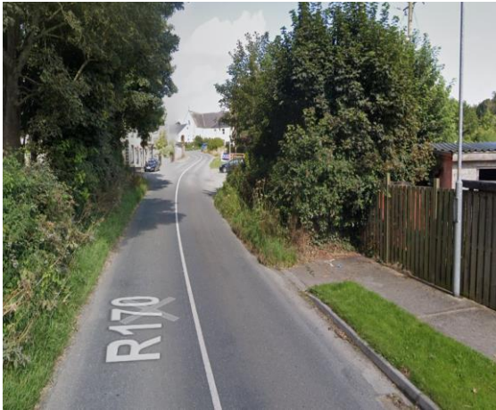
Dromin Footpath prior to works
